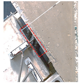
Observed Behavior: ED bar buckling and dowel plate yielding at failure
