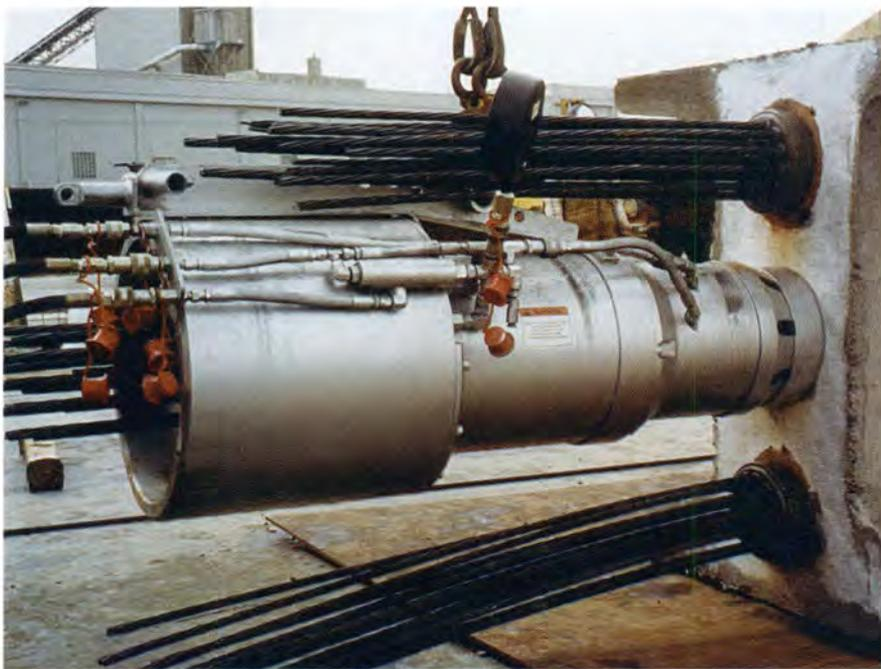
Fig. 10. Middle tendon during post-tensioning.
