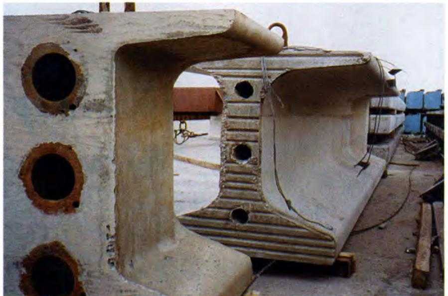
Fig. 9. Match-cast joint surface.
