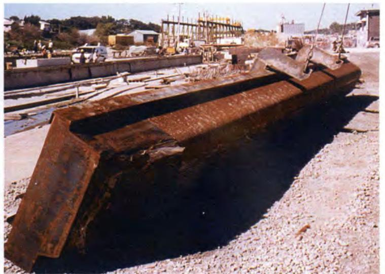
Fig. 12. Steel form for tapered anchorage zone.
