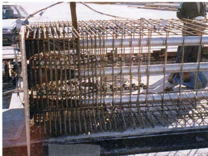
Fig. 5. The general zone reinforcing cage (Detail 1).
