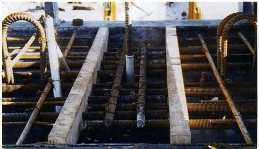
Fig. 18. Method for aligning continuity reinforcement.
