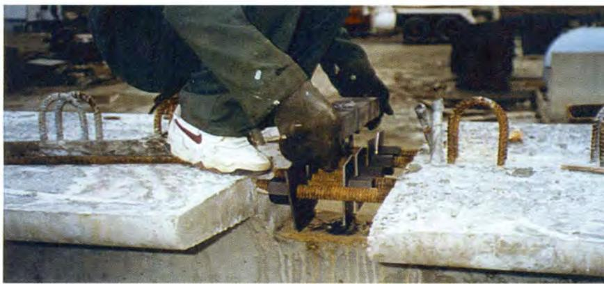
Fig. 19. Placement of rectangular steel bar.
