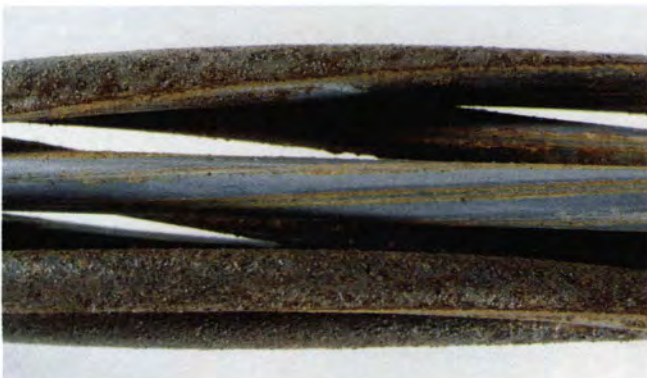
Photo 8. Strand surface before cleaning.
