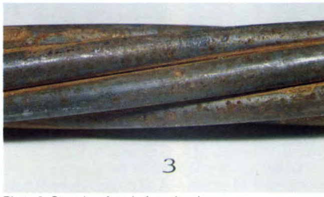
Photo 3. Strand surface before cleaning.
