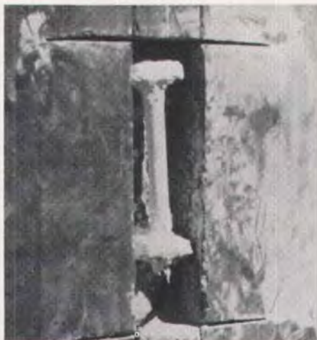
Fig. 3. Installed strain gauge after concrete casting.
