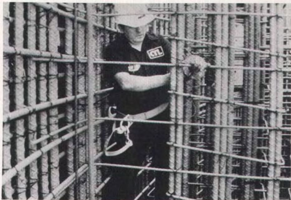
Fig. 4. Installation of gauges before concrete casting.
