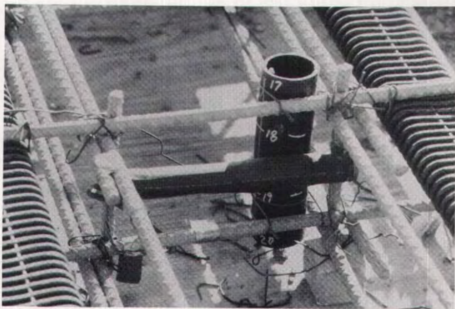
Fig. 5. Installed gauges at precasting plant.
