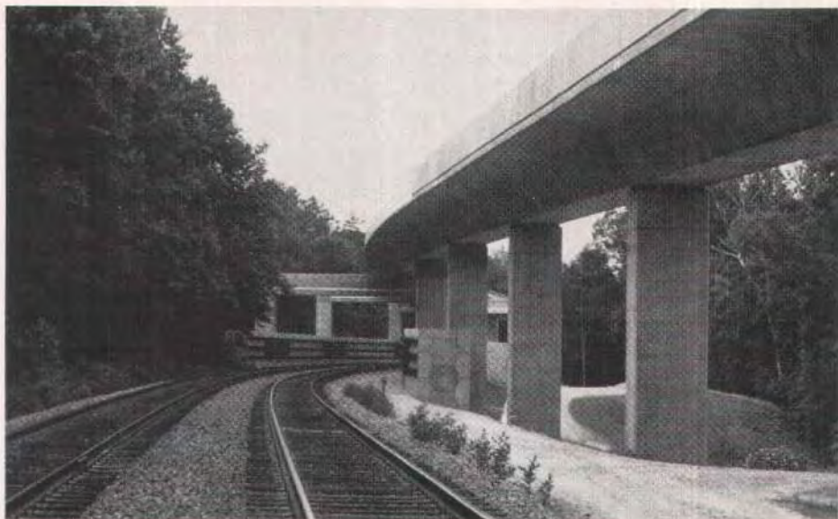
Its track in place, the completed superstructure curves gracefully above and alongside the heavy rail track.
