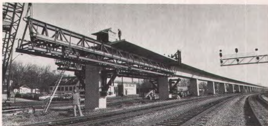
Overall view of span by span construction of precast superstructure.
