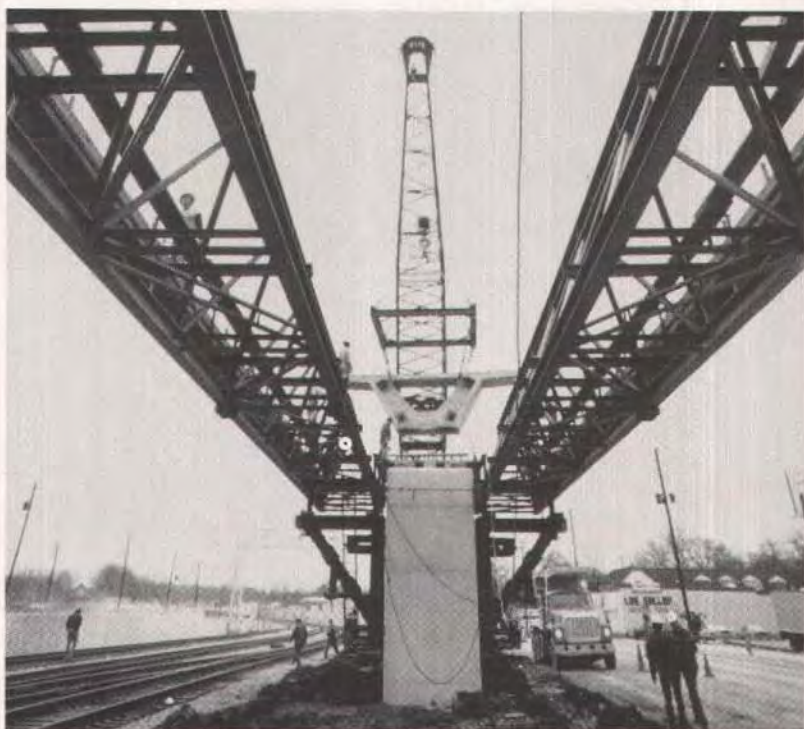
Segment being placed on twin triangular trusses.
