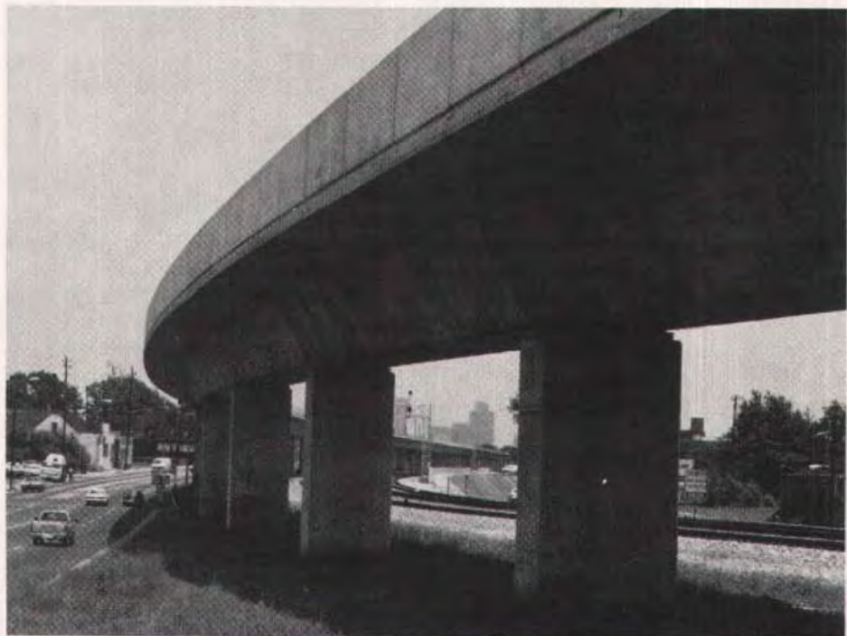
The first elevated structure runs parallel to a busy thoroughfare and railway line. Precast segmental construction with triangular trusses allowed construction to continue without interruption of traffic.
