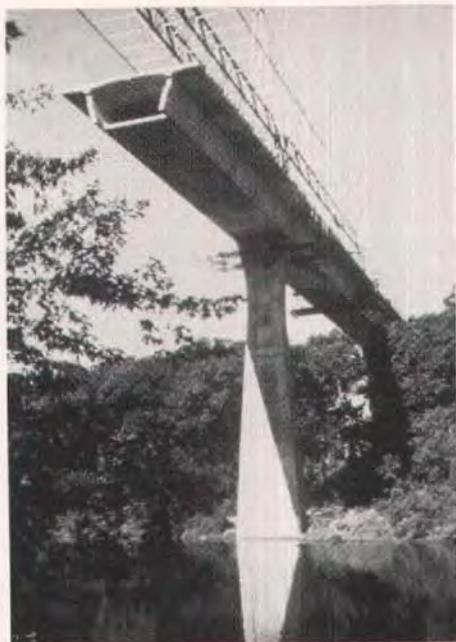
Fig. 1a. Balanced cantilever erection using a launching truss.
