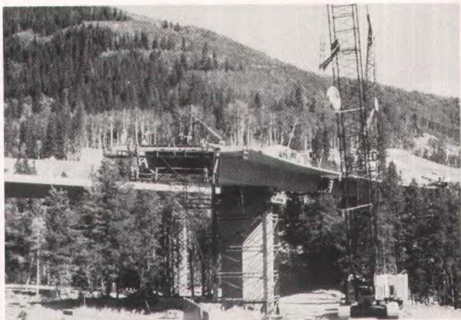
Fig. 1b. Precast segmental box girder bridge being erected in balanced cantilever fashion using a crawler crane.
