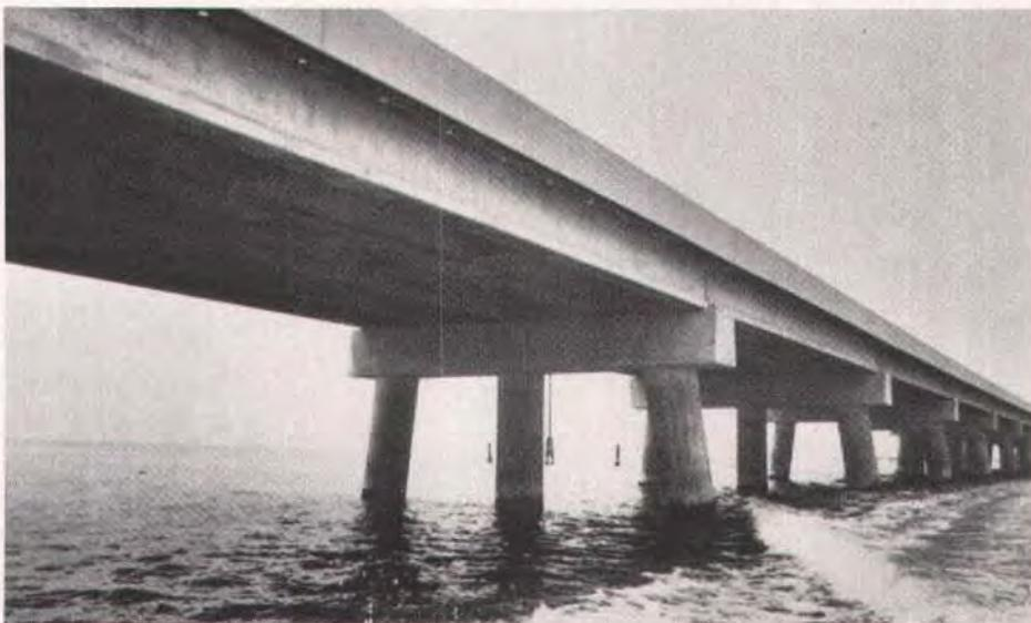
*Fig. 10. A total of 178 65-ft (19.8 m) monolithically precast spans were used in the low-level approaches of the bridge. The piers are made up of three 54-in. (1372 mm) diameter cylindrical precast piles and a precast cap.*
