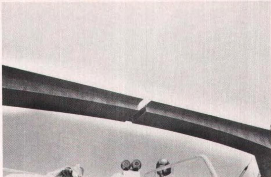
*Fig. 25. Gap at centerline of main 400-ft (120 m) span ready for cast-in-place closure. Approximately two precast segments per 12-hour day were erected.*
