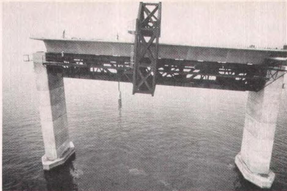
*Fig. 29. Approach span with all segments in place on truss. After pier segment is placed the final post-tensioning will be done and truss moved to next span.*
