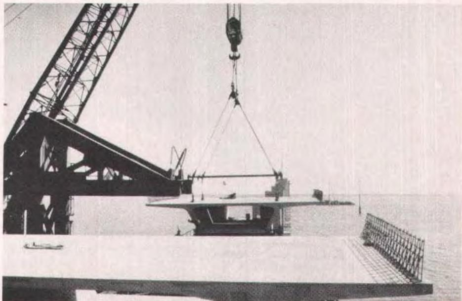
*Fig. 30. Placing precast segment on erection truss. All segments made with transverse grooves in deck with steel ties. No additional surfacing is necessary.*
