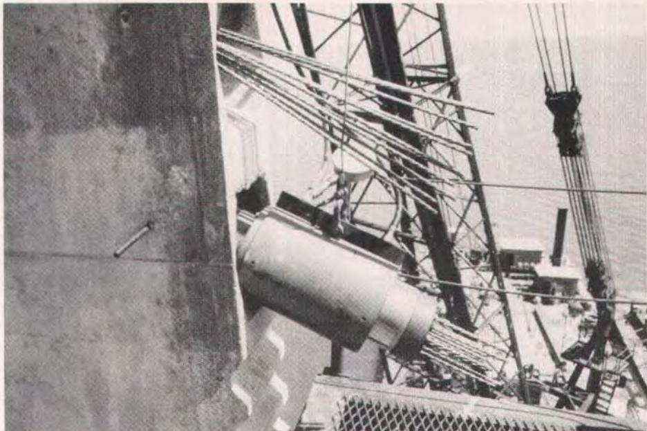
*Fig. 22. Hydraulic jack being used to tension tendons for erection stresses.*
