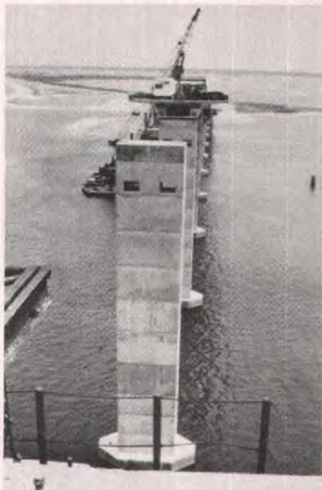
*Fig. 16. The top segment of each pier contained rectangular blockouts to support the steel erection trusses for span-by-span erection.*
