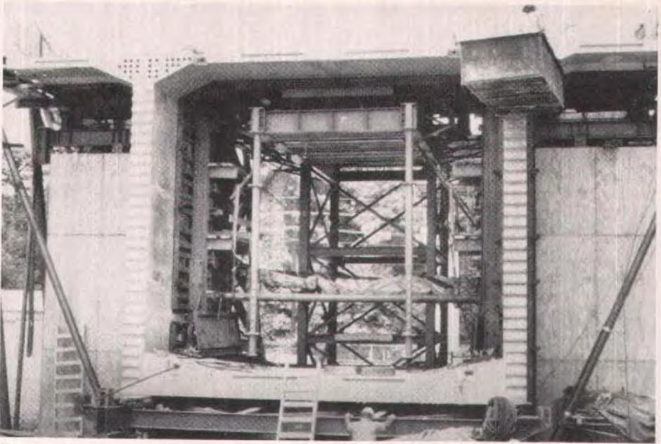
*Fig. 11. Precast segment ready for match casting in forms at Mandeville plant. Note multiple keys.*
