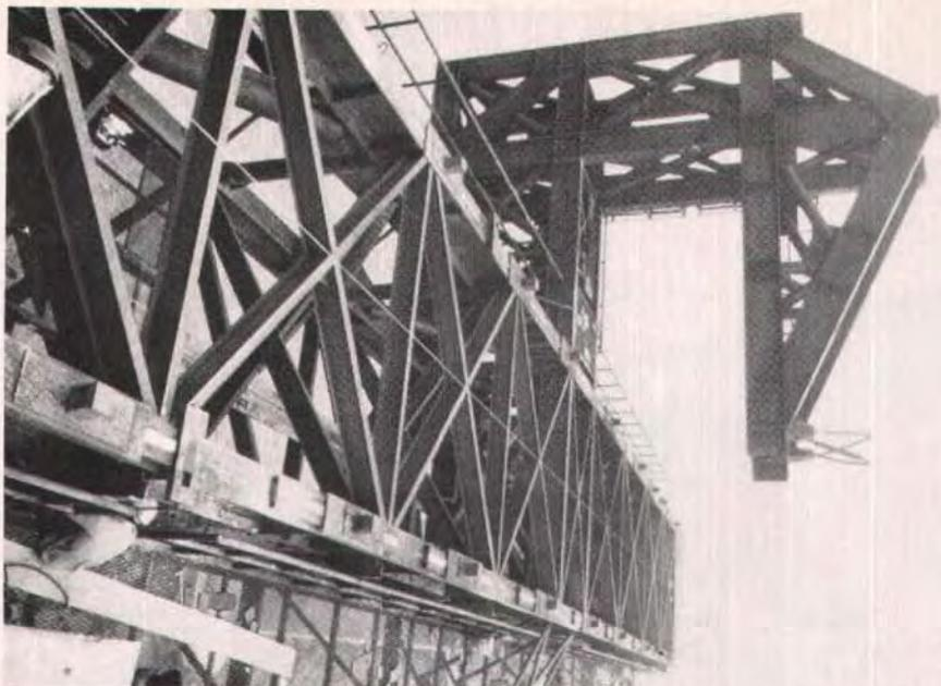
*Fig. 27. Closeup of erection truss used for span-by-span construction of 118-ft (36 m) high level approaches.*
