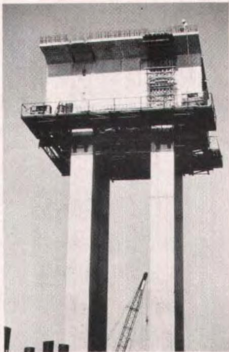
*Fig. 18. Pier segments, precast and cast-in-place, ready for adding precast box segments.*
