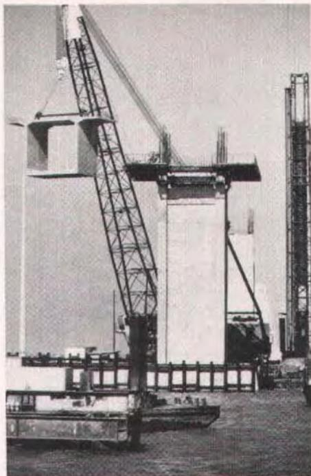
*Fig. 17. Barge-mounted crane lifting pier segment for main span. Note that main piers were twin walled.*
