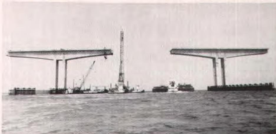
Fig. 24. *Balanced cantilever construction in progress on 400-ft (120 m) precast main span and 211-ft (64.3 m) side spans. Note that segments vary in depth from 21 ft 5 in. (6.5 m) at the piers to 7 ft (2.1 m) at midspan.*
