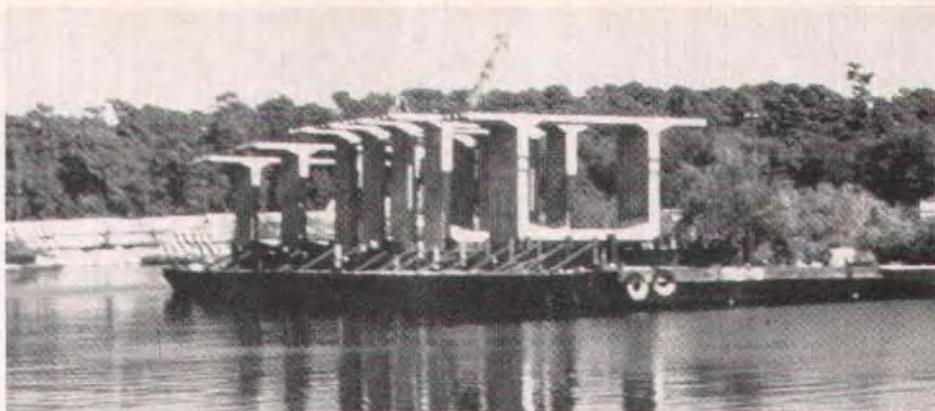
*Fig. 13. Precast segments for 400-ft (122 m) main span were barged 150 miles (240 km) to construction site.*
