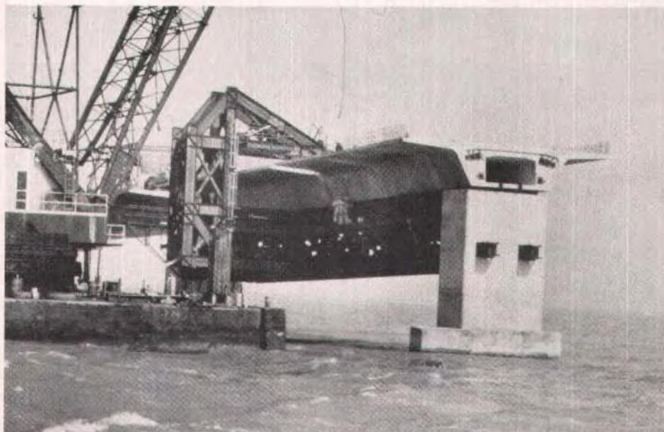
*Fig. 28. A large steel truss hanger is used to move truss, which supports segments until post-tensioning is complete. Note blockouts in piers to support truss.*
