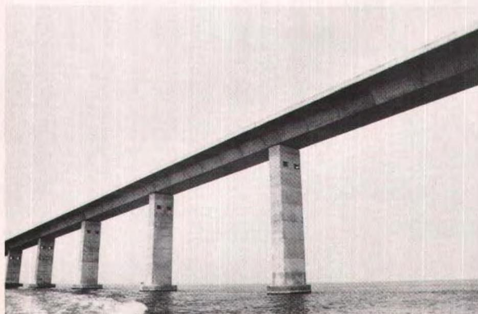
*Fig. 32. Approach spans complete and ready for casting the safety shape parapet, the last step in erection procedure.*
