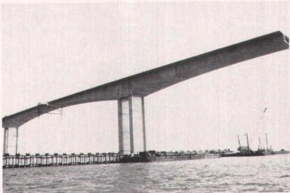
*Fig. 26. Main spans almost complete. Structure is now ready for adjacent spans which were erected by span-by-span method.*
