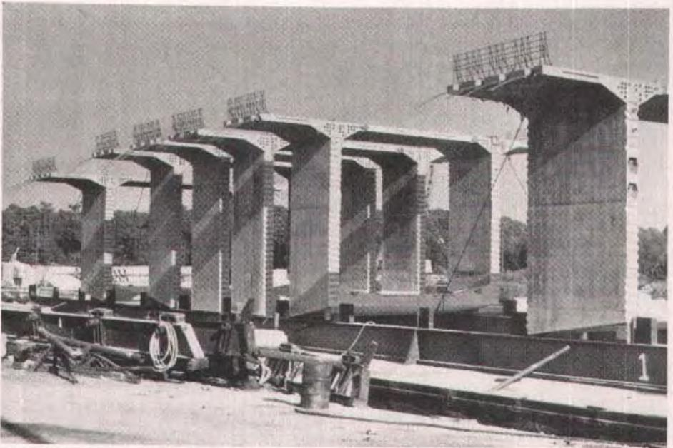
*Fig. 12. Several variable depth, match-cast segments for main spans are being air cured prior to shipment to bridge site.*
