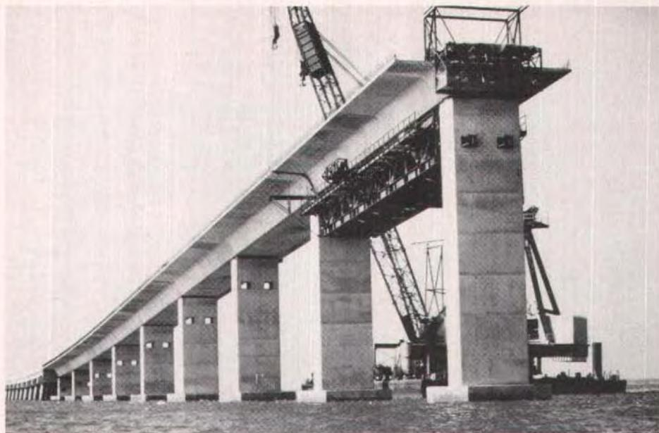
*Fig. 31. Large barge-mounted crane ready to move erection truss to next span.*
