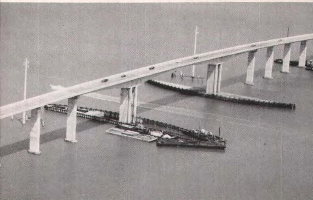
*Fig. 3. Dauphin Island Bridge in service. The center span is 400 ft (122 m) with a vertical clearance of 85 ft (26 m) to allow small ships and sea craft to pass. The two side spans are 211 ft (64.4 m).*
