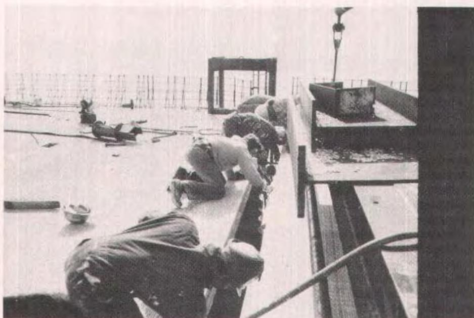
*Fig. 21. Workmen coating faces of precast segments to insure good bond between match-cast segments. Note reinforcing bars along box edges for cast-in-place safety shape parapet.*
