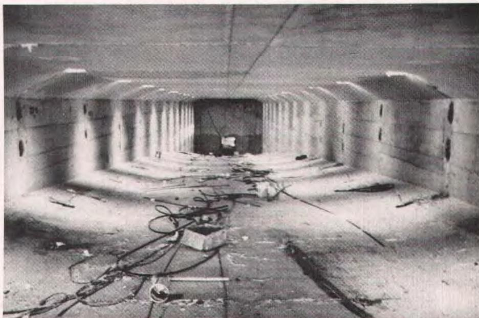
*Fig. 23. View inside box looking toward main span pier diaphragm. The variable depth of the box, 7 ft (2.13 m) at the midspan to 21½ ft (6.56 m) at the piers, is noticeable. Empty space can be used for inspection purposes.*
