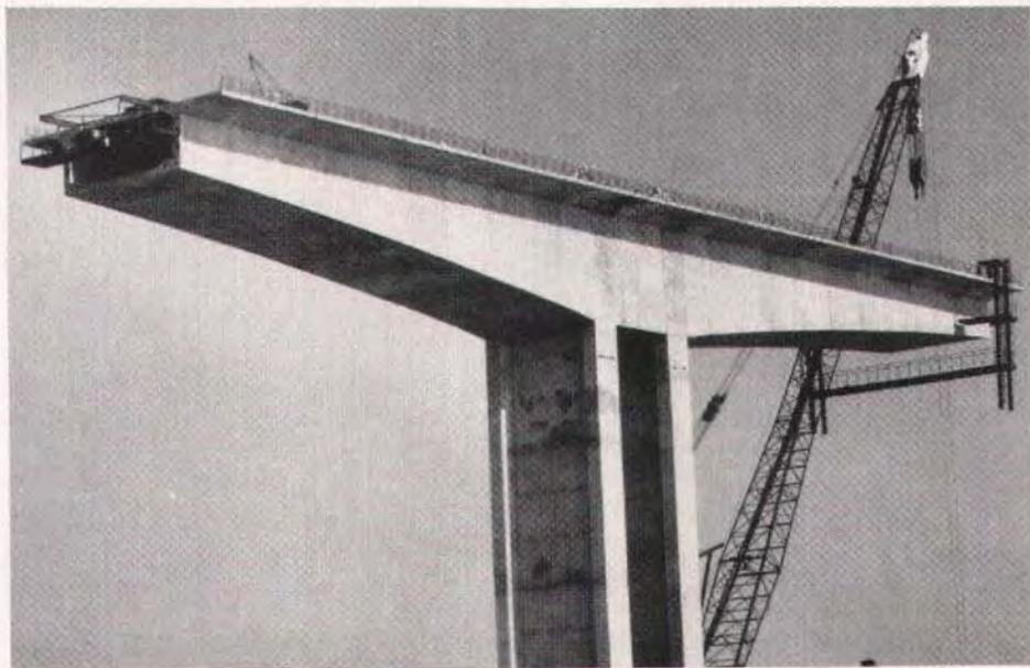
*Fig. 19. One of two main piers supporting balanced cantilever of precast box segments.*
