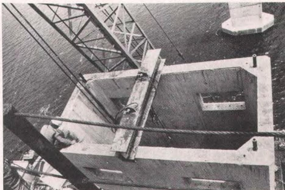
*Fig. 14. Pier segments for all precast segmental approach spans were precast. The dimensions are 16 x 8 ft (4.88 x 2.44 m) with 10-in. (254 mm) thick walls.*
