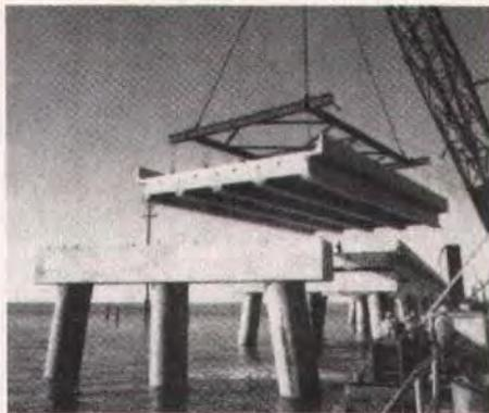
*Fig. 9. Monolithically precast 65-ft (19.8 m) spans each consisted of five girders, a deck, and two safety shape parapets. These units weighed 270 tons (245 tonnes) each.*
