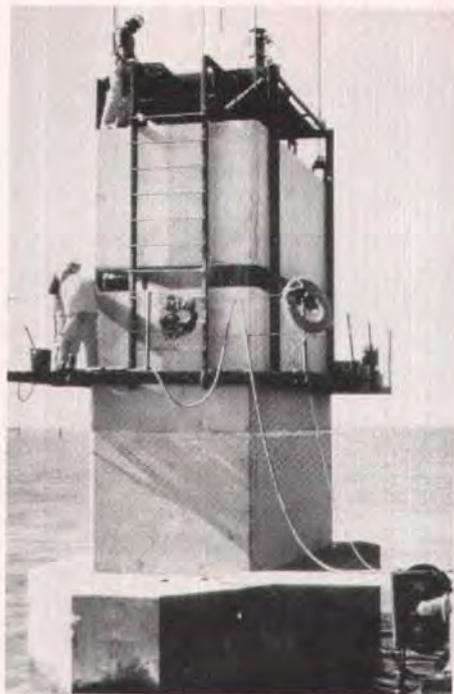
*Fig. 15. Workers' platform, which surrounded the piers, was jacked up as the pier progressed upward to provide access to joints where epoxy was used.*
