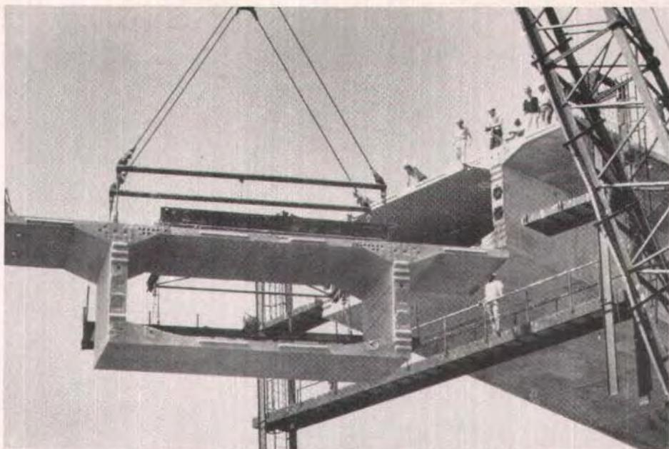
*Fig. 20. Barge-mounted crane lifting precast segment to attach to cantilever. Shallow depth of box indicates span is nearly complete.*
