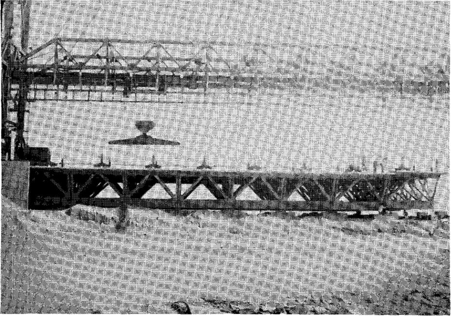
Fig. 29. Erection of first span of bridge. Note that embankment under the first span is temporary and used only as a precautionary measure.
