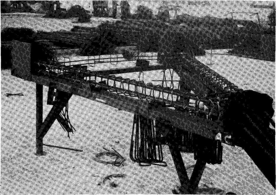
Fig. 15. Fabrication of triangle reinforcement cage.
