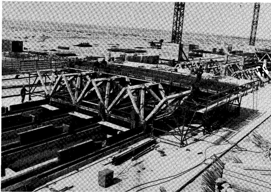
Fig. 25. Precast triangles on jigs positioned in casting bed (courtesy of Bouygues).
