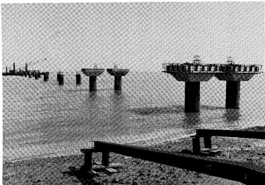
Fig. 9. Typical twin pier shafts (courtesy of Bouygues).
