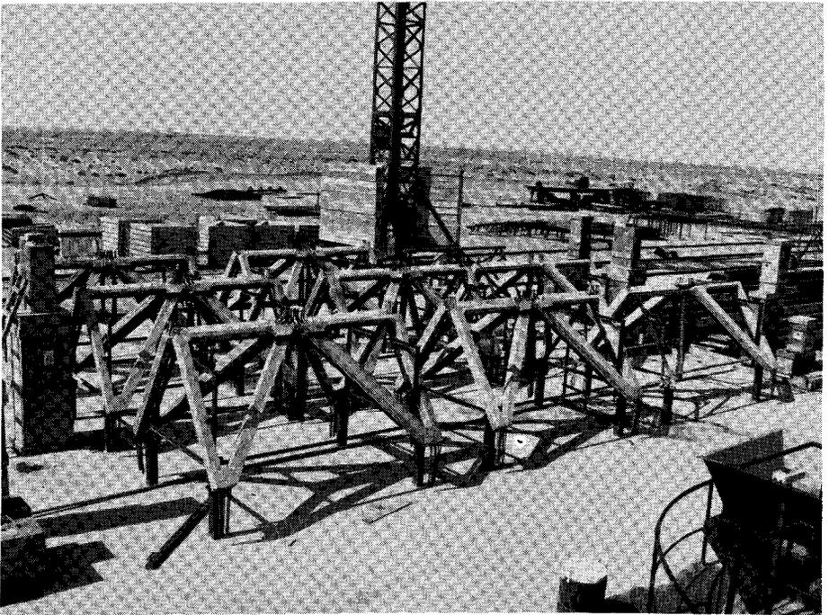
Fig. 24. Precast triangles positioned on jigs (courtesy of Bouygues).
