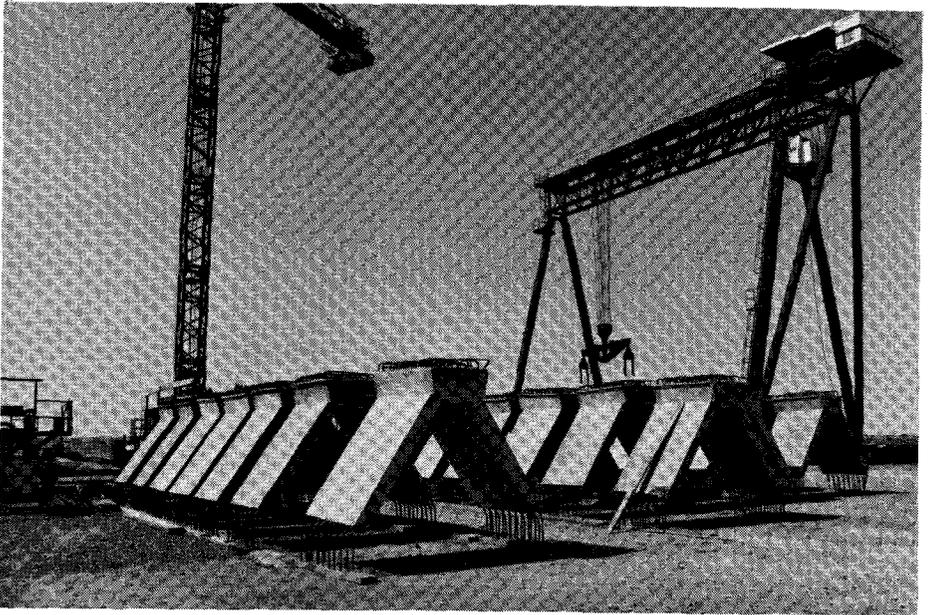
Fig. 20. Pier segment diagonals in storage yard (courtesy of Bouygues).
