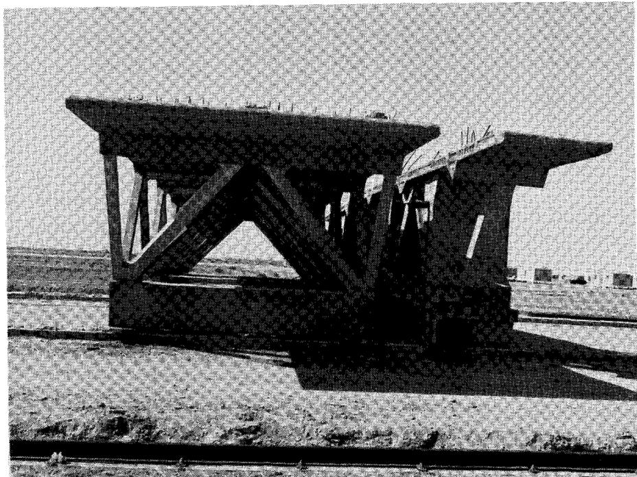
Fig. 10. Typical segment and pier segment (courtesy of Bouygues).
