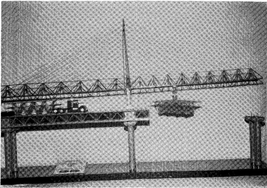
Fig. 4. Construction stage model of Bubiyan Bridge.
