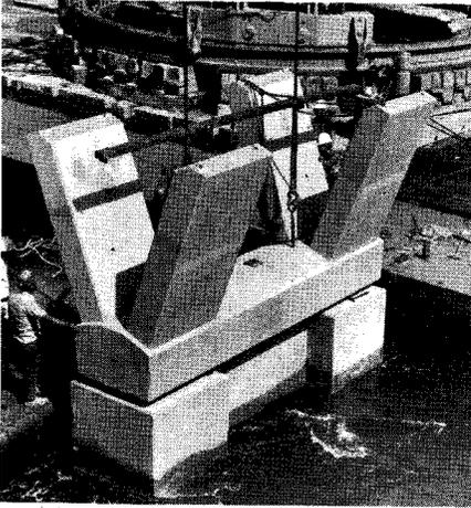
Fig. 2. Placing precast V-pier on cap (Long Key Bridge).
