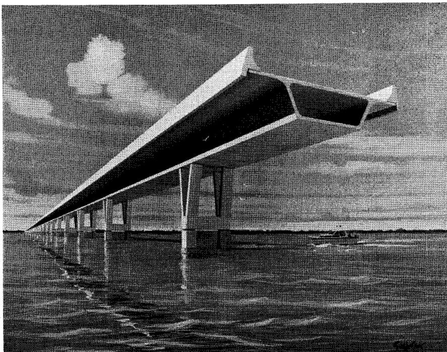
*Fig. 1. Rendering of Long Key Bridge in Florida. The successful bid used precast segmental span by span construction with precast V-piers and drilled shaft foundations. (Courtesy: Figg and Muller Engineers, Inc.)*
