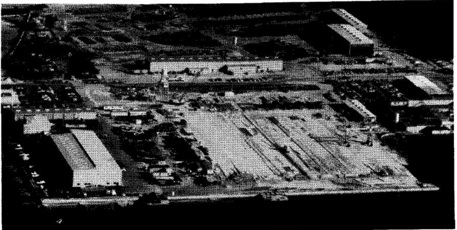
Fig. 4. Casting yard in Tampa, Florida, for Seven Mile Bridge.
