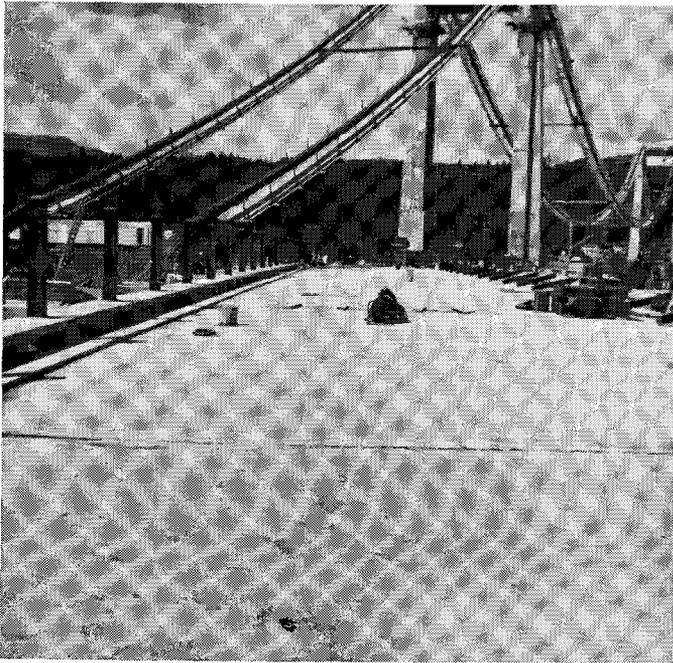
Fig. 8—Segmental Units in Casting Bed
