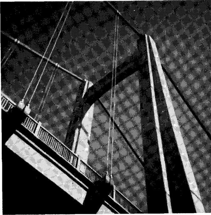
Fig. 10—Main Cable and Suspenders
