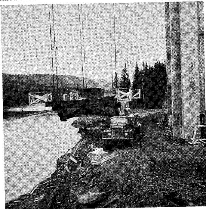
Fig. 14—Segmental Unit on Low Bed
