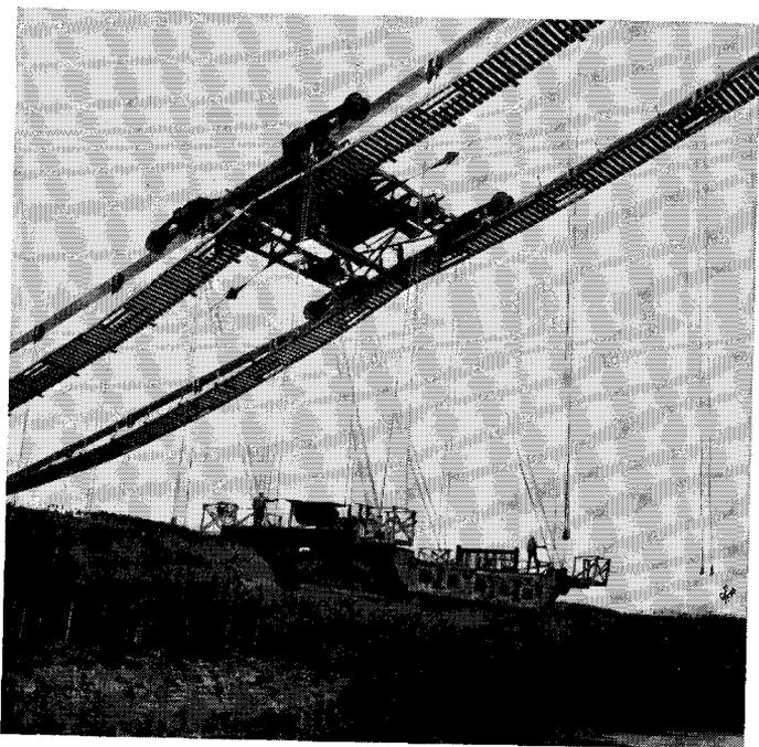
Fig. 15—Erection of Segmental Units
