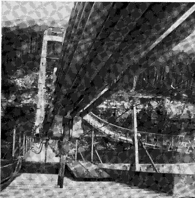
Fig. 9—Main Cable and Suspenders
