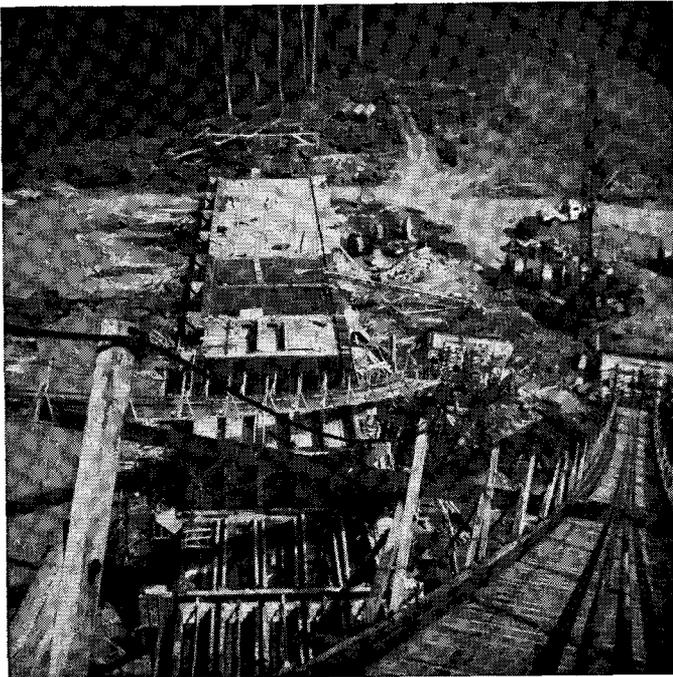
Fig. 7—Segmental Units in Casting Bed
