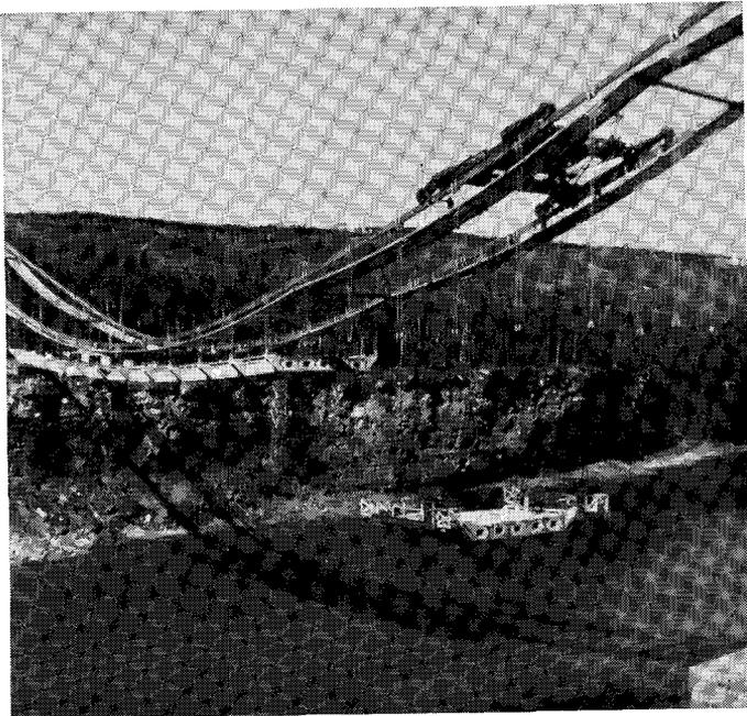
Fig. 16—Erection of Segmental Units
