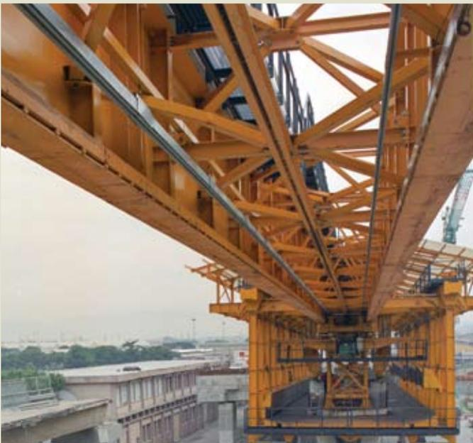
**Figure 5.** Lateral bracing of a single-upper-beam gantry in a movable scaffolding system configuration connects the plate girders along their entire length.
