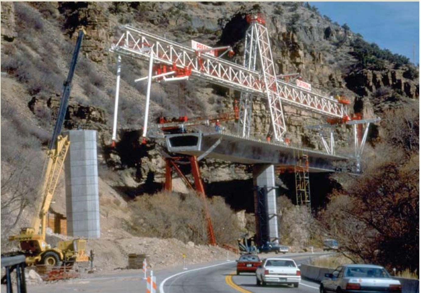
**Figure 11.** This single-upper-truss gantry is equipped with a deviation tower. Photograph courtesy of HNTB archive.
