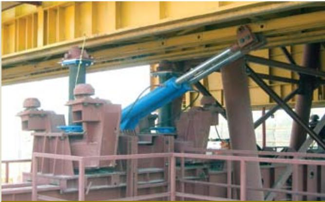
**Figure 4.** The launch cylinders of a twin-lower-beam gantry are shown in the raised configuration for segment assembly.
