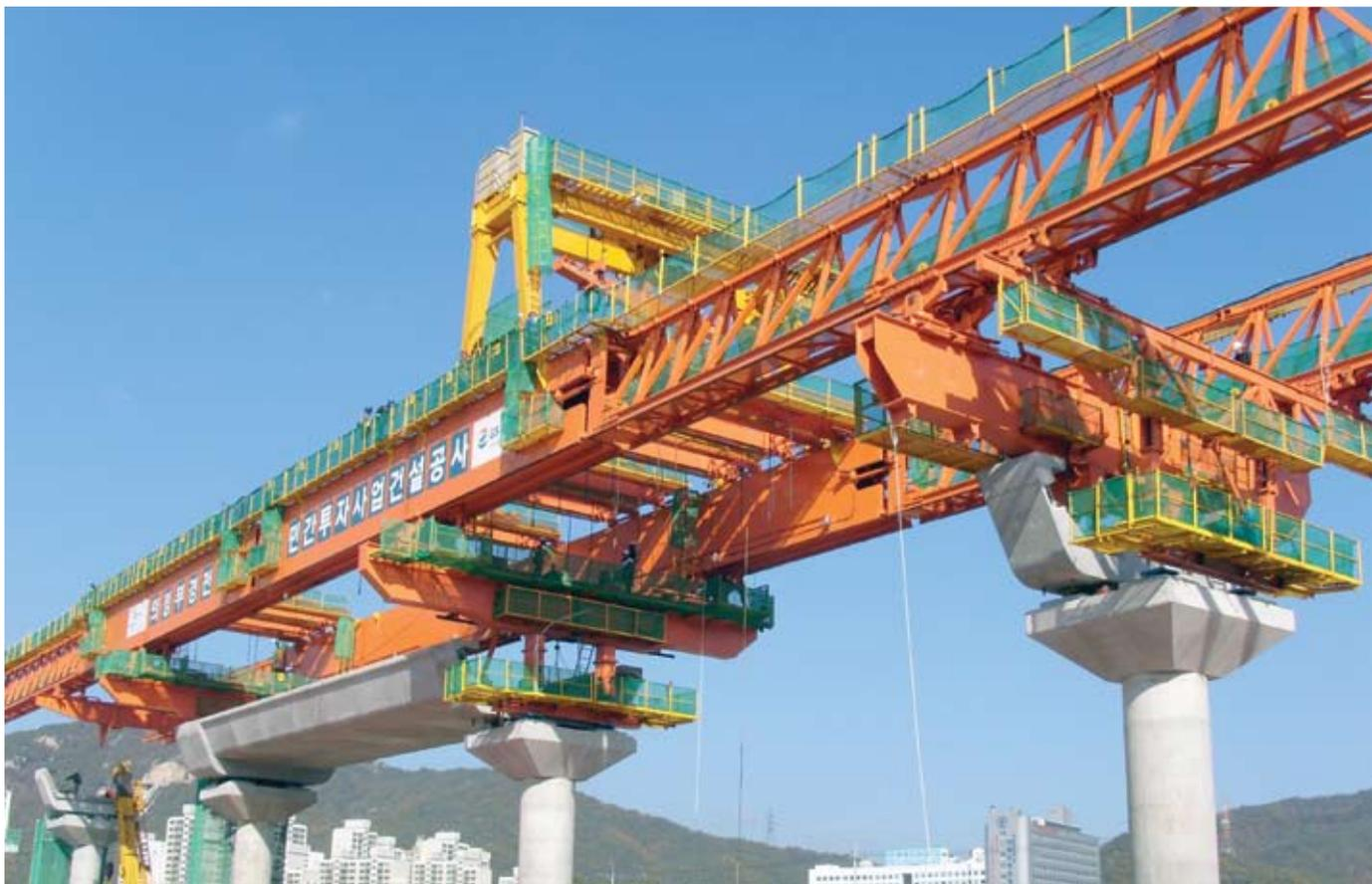
**Figure 3.** This shows a twin-upper-beam gantry with support cross beams. Photograph courtesy of NRS.
