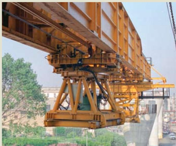
**Figure 7.** The friction launchers are suspended from the main girder.
