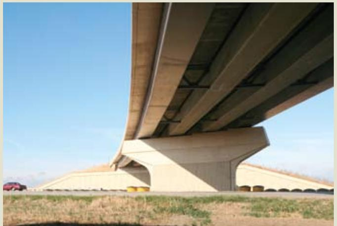
**Figure 6.** The Arbor Road Bridge in Lincoln, Neb., is a two-span, horizontally curved, precast concrete-girder bridge with a skew of 31 degrees and a central angle of about 3 degrees.
