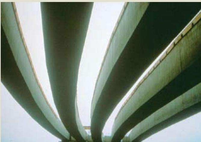
**Figure 3.** The curved, precast, post-tensioned concrete box girders used for the Philadelphia Airport renovation are in their final position. Courtesy of Joseph Nagle, Schuylkill Co.
