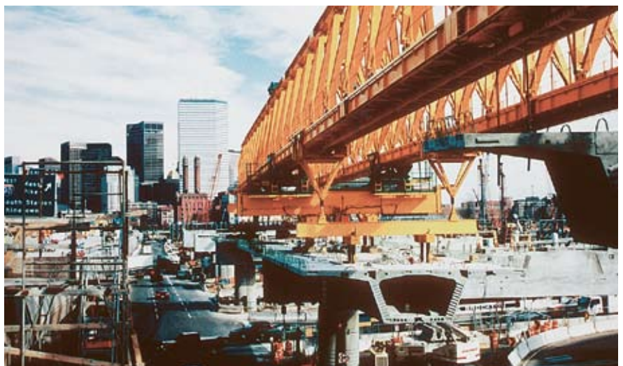
Fig. 5. Self-launching overhead gantry.
