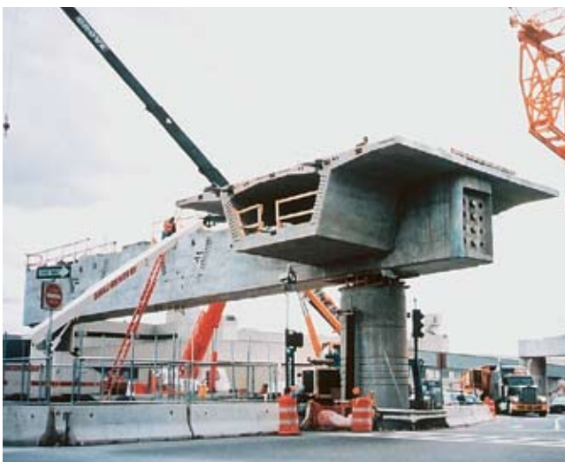
Fig. 9. Straddle bent with precast segments.
