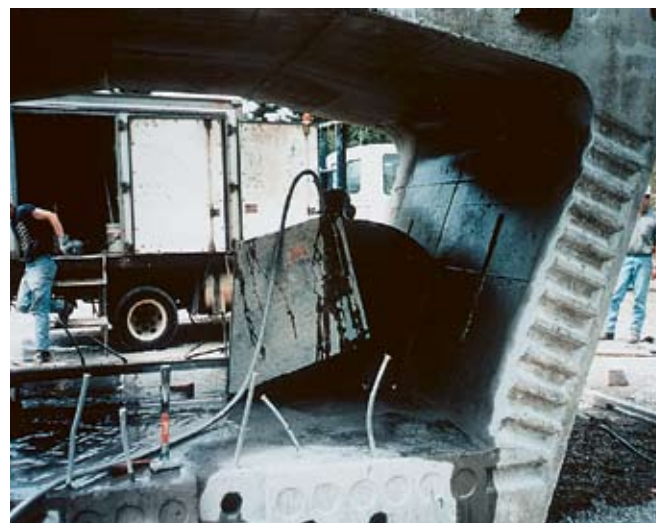
Fig. 10. Saw cutting of segment.
