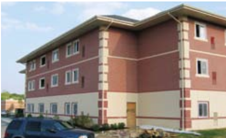
Eight-four unit assisted-living facility built to withstand an F-4 tornado. Photo: Dukane Precast Inc.
