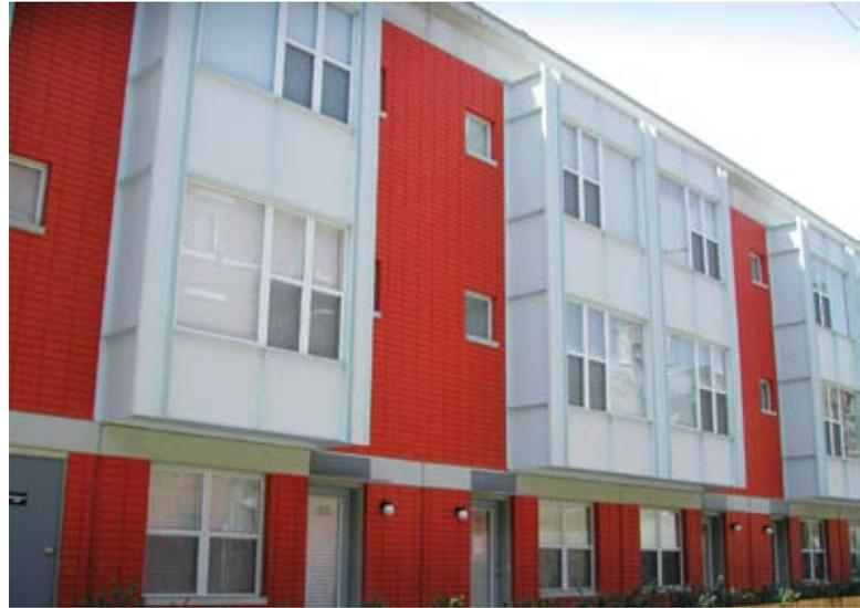
*Arcadia Place in Chicago, designed by Landon/Bone/Baker Architects and developed by Dubin Residential, features stacked-bond patterned precast concrete wall panels, smooth panels with reveals, garage headers and precast concrete parapets provided by Prestress Engineering Corp. in Prairie Grove, Ill.*
