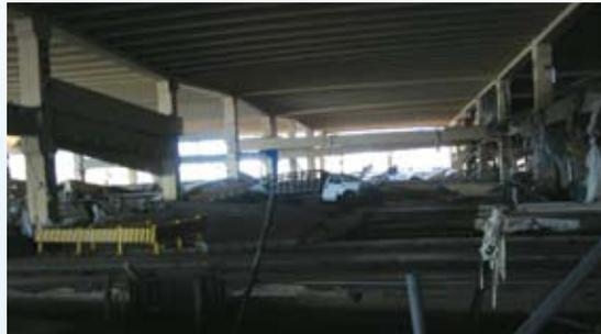
*Much of the damage done to precast concrete parking structures along the Gulf Coast by Hurricane Katrina was caused by the high storm surge, which flooded the structures and caused double tees to be pushed off their supports. Otherwise, the material performed well.*
