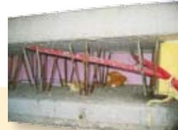
Radiant tubing cast into the Fortified floor panels. Photo: Dukane Precast Inc.
