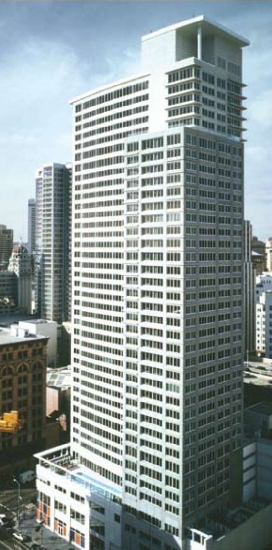
The Paramount's use of a precast hybrid, moment-resisting frame as part of its structural system is that it creates a restoring force provided by its elastic, post-tensioned strands that rights the building following a seismic event. Architect of Record: Kwan Henmi, Architecture/Planning; Photo: David Wakely Photography.
