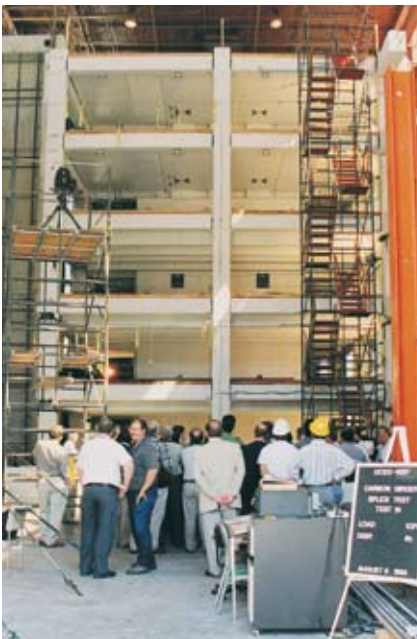
Rigorous tests performed on an experimental structure proved the success of the PRESSS program's connection technology.
