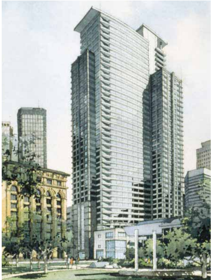
The 680 Mission Apartments building, a 39-story skyscraper in San Francisco, currently is under construction using a precast concrete hybrid moment-resistant frame for structural resistance. The structural components also serve as architectural cladding. Rendering: Elkus/Manfredi
