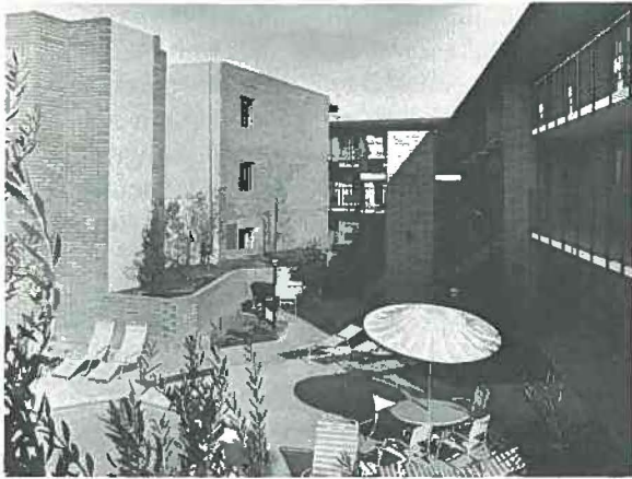
Masonry walls are ideal for apartment construction. They provide a barrier against the spread of fire while maintaining structural integrity.
