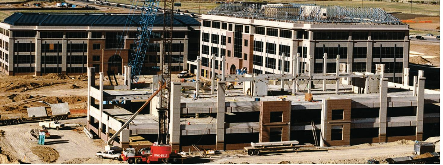
Quality control extends to installing engineered components, such as precast prestressed concrete panels, beams, or other components. Using certified producers creates better tolerances that minimize field adjustments, while certified erectors increase safety.
