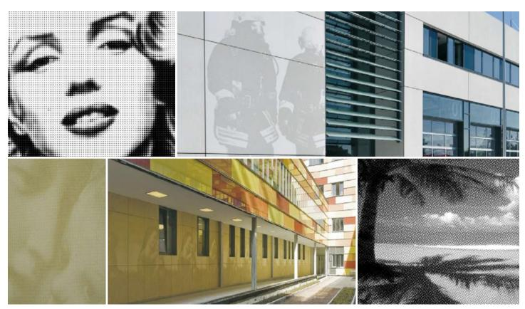
Photo concrete. Different than photo-engraved concrete, the image appears to be printed onto the concrete.
