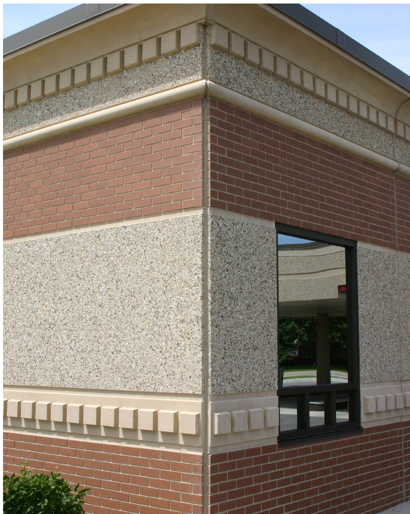
The Wells Federal Bank in Mankato, MN provides an example of how exposed aggregate can work with other precast concrete finishes to provide a unique, classic look. (Image Credit: Wells Concrete)
