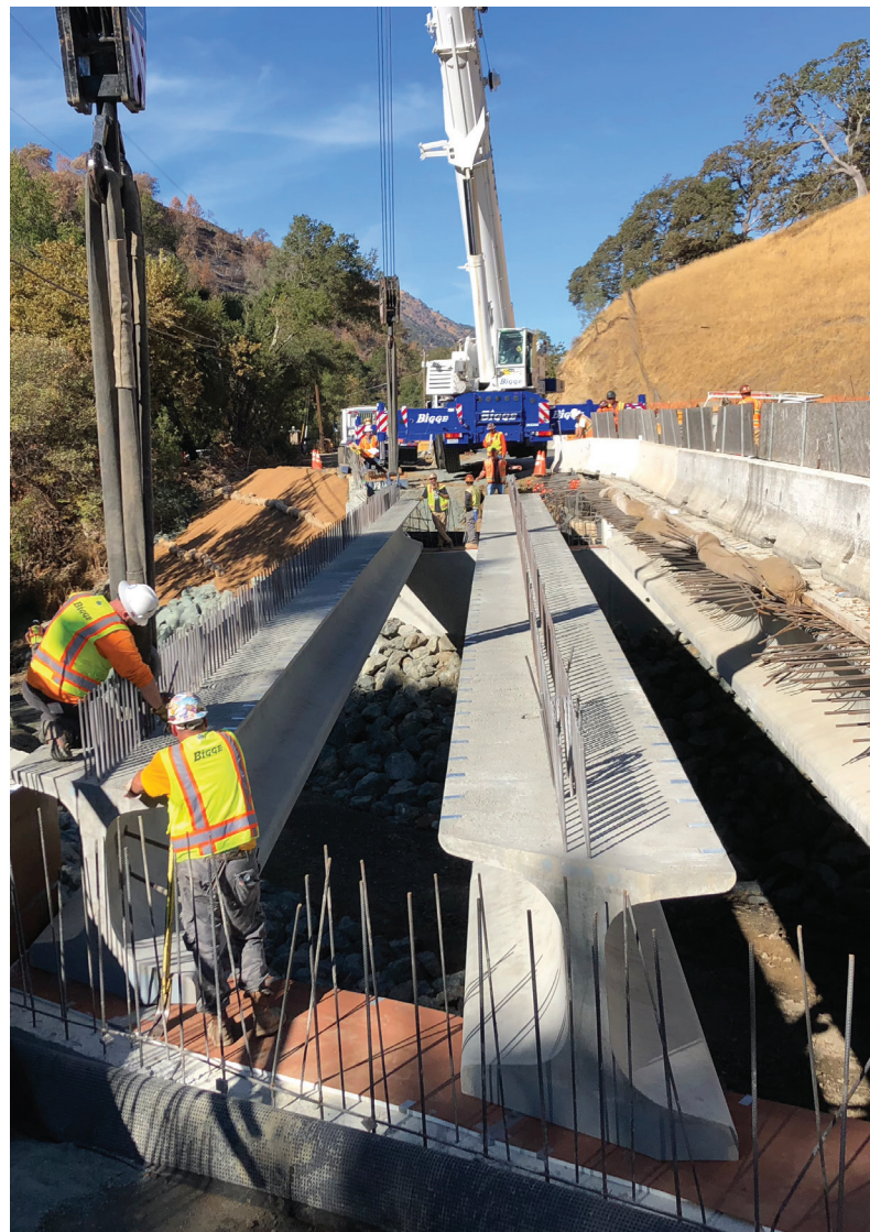
Con-Fab installed the six girders for the Marsh Creek Road bridge replacement project near Clayton, Calif., in two stages. The second stage of girder erection on the accelerated bridge construction project is shown here. Courtesy of Con-Fab.
