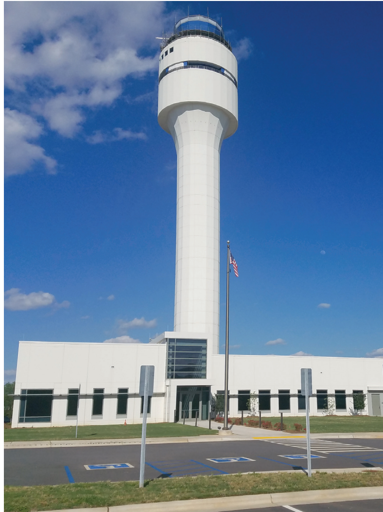
Gate provided precast concrete for the new airport traffic control tower in Charlotte, N.C. It's the second tallest airport traffic control tower in North America. Courtesy of Gate Precast.
