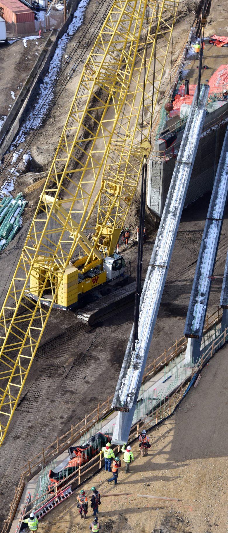
Erecting the extremely large girders for the Interstate 15 Technology Corridor project in Utah County, Utah, required a complicated two-crane placement. Courtesy of Forterra Structural Precast.
