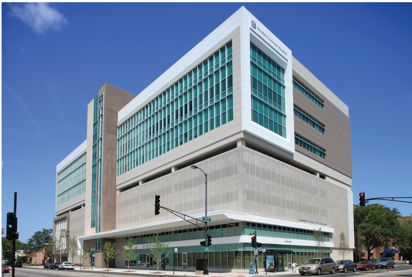
Spancrete provided precast concrete for the Foster Medical Pavilion, part of Swedish Covenant Hospital in Chicago, Ill. The facility took seven weeks to install, and precast concrete reduces vibrations in the medical offices from the parking structure. Courtesy of Spancrete.
