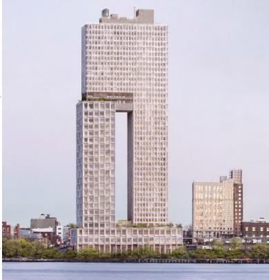
This rendering shows the Domino Sugar Refinery redevelopment project in Brooklyn, N.Y. Gate Precast Co. teamed up with Oak Ridge National Laboratory to create the forms for the window panels in the 42-story, mixed-use 260 Kent Avenue structure—the tallest building in the project—using 3-D printing. Rendering by COOKFOX Architects.
