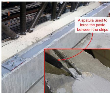
**Figure A10.** Filling the groove with paste adhesive.
