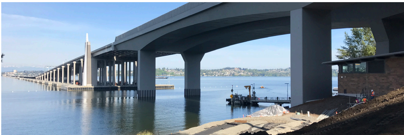
Construction of the Evergreen Point Floating Bridge faced challenges such as geometric height constraints of the travel way to the lake level. Courtesy of BergerABAM.
