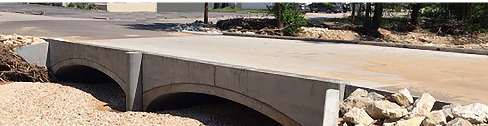
The Dyer Street Road bridge in Waynesville, Mo., used County Materials’ ArchCast system to elevate a low-water crossing. The Roubidoux Creek can go from its typical 1 ft (0.3 m) of water to as much as 21 ft (6.4 m) when it floods. The stream bottom is in the process of reshaping. The low-water crossing caused fill to back up upstream of the new bridge. Photo courtesy of County Materials Corp.
