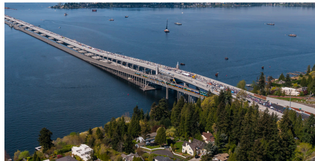
The Evergreen Point Floating Bridge uses 77 precast concrete pontoons to support Washington State Route 520 across Lake Washington in Seattle. Courtesy of Washington State Department of Transportation.
