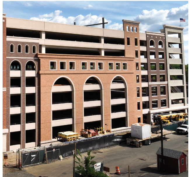
The 3400-vehicle parking structure for the MGM Springfield resort in downtown Springfield, Mass., uses a total–precast concrete structural system. Courtesy of MGM Springfield (photo by Mark M. Murray).
