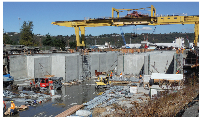
The precast concrete pontoons for new cruise ship berths in Juneau, Alaska, were fabricated in Concrete Technology Corp.'s dry dock in Tacoma, Wash., and towed to Juneau, Alaska. Courtesy of BergerABAM.
