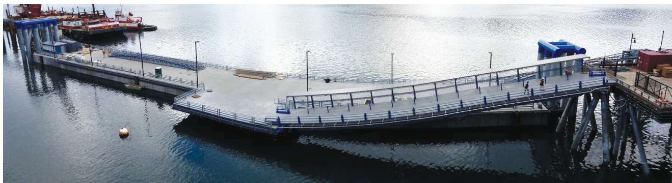
The north precast concrete pontoon was designed to accommodate post-Panamax-sized cruise ships in Juneau, Alaska. Courtesy of Monica Blanchard—Manson Construction Co.
