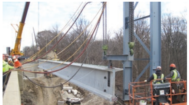
The substructure of the Interstate 90 bridge over the Fox River in Elgin was constructed under the existing bridge. Courtesy of Scott Eshleman.
