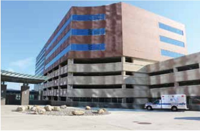
The Stamford Integrated Care Pavilion/Medical Office Building in Stamford, Conn., uses precast concrete to combine open medical office areas with a shear-wall system for parking. Photo courtesy of Blakeslee Prestress Inc.
