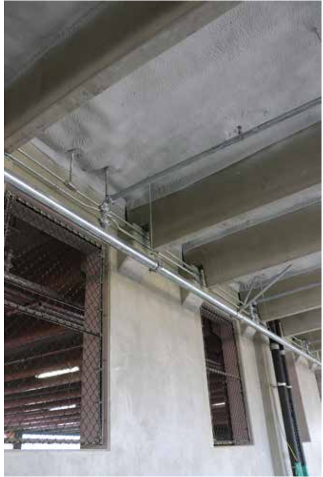
The lateral design of the Stamford Integrated Care Pavilion/Medical Office Building used precast concrete litewalls for the parking levels and a precast concrete moment-frame system for the office levels to provide large open-floor plates with minimal columns and no shear walls. Photo courtesy of Blakeslee Prestress Inc.
