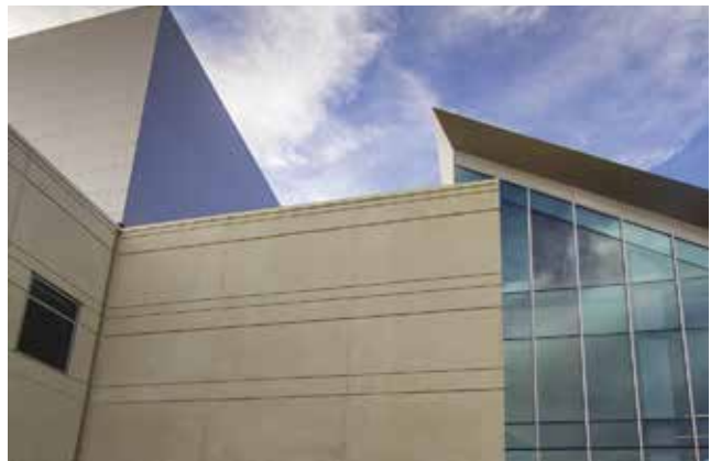
The insulated wall panels provide an R -value of 12 and helped the building receive LEED silver certification. Courtesy of AECOM.
