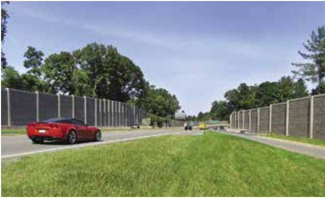
The Route 29 and Route 250 interchange in Charlottesville, Va., uses Smith-Midland's SoftSound concrete for noise barrier walls that have finishes designed to go with the look of the area. Courtesy of Smith-Midland Corp.
