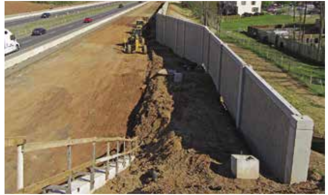
Designed to complement nearby historic Chapman's Mill, Va., the precast concrete sound walls for a highway widening project were provided by Smith-Midland. Courtesy of Smith-Midland Corp.
