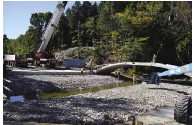
Workers erect precast concrete arches for bridges on Warden Avenue in Markham. Courtesy of Armtec LP.
