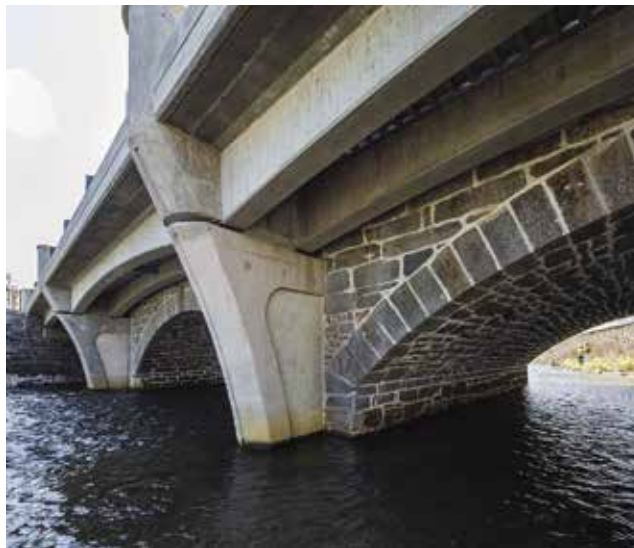
Precast concrete was used to rehabilitate this 1890s stone arch bridge that had deteriorating sidewalks in Tamaqua, Pa. Courtesy of John Baer/Building Images Photography.
