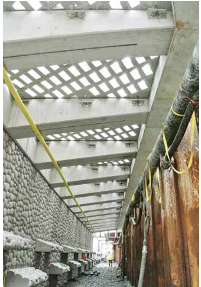
Precast concrete Z-shaped superstructure segments are the backbone of the new Elliott Bay Seawall reconstruction project's cantilevered sidewalks in Seattle, Wash.
