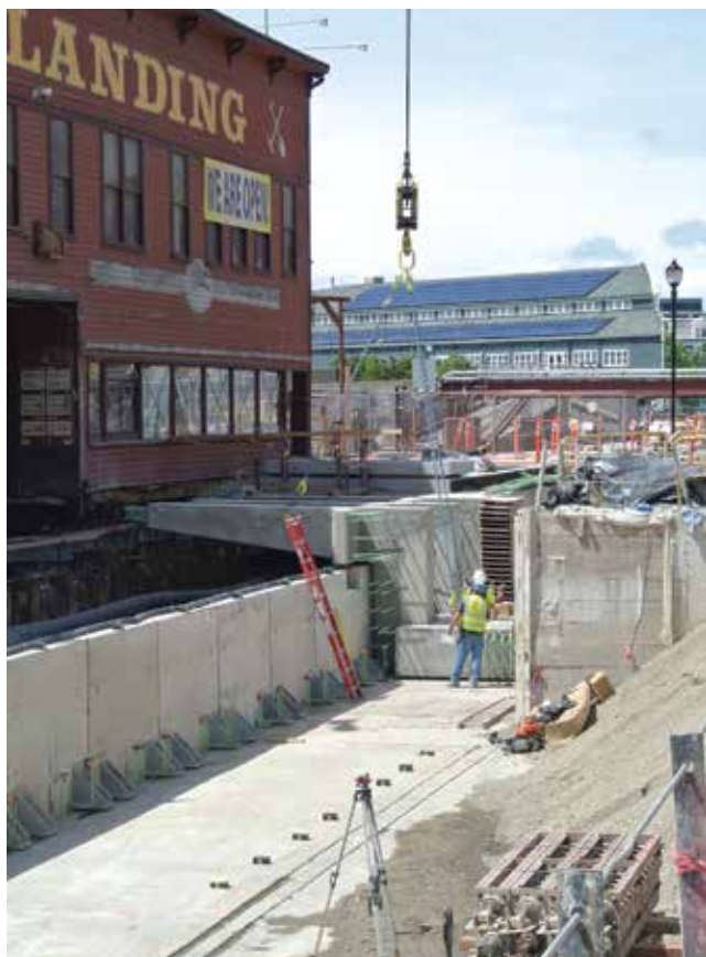
The closure wall behind the Z-shaped panels is being assembled near Waterfront Park in Seattle, Wash. Oldcastle Precast is supplying 400 precast concrete Z-shaped superstructure segments for the Elliott Bay Seawall reconstruction project. Courtesy of City of Seattle.
