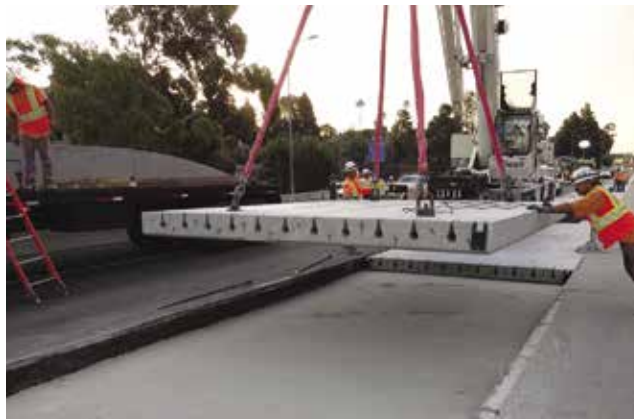
A crane lowers a precast jointed concrete panel into place during the repair of US Route 101 in California.
