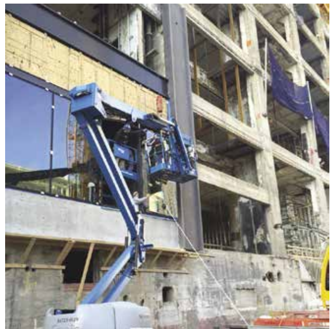
Precast concrete was used to reclad the eight-story building at 34 S. 11th St. in Philadelphia as part of the East Market rehabilitation project.
