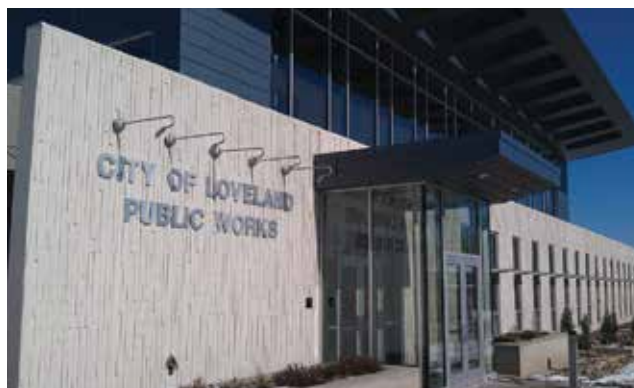
Stresscon used a decorative formliner for the new city of Loveland public works main office building entrance in Colorado. In addition to aesthetics, precast concrete also provided energy savings, durability, quick erection, and low maintenance. Courtesy of EnCon United.
