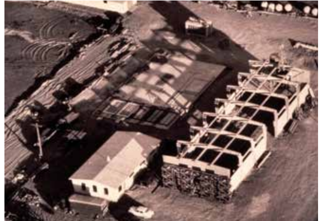
After returning from a trip to Europe to tour prestressed concrete plants, Concrete Technology Corp. constructed the first prestressed concrete building anywhere in the United States. This aerial shot shows the building, which is used for manufacturing precast concrete panels. Courtesy of Concrete Technology Corp.
