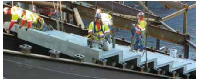
Workers erect a panel for Levi's Stadium in Santa Clara, Calif. Courtesy of © Todd Quam.
