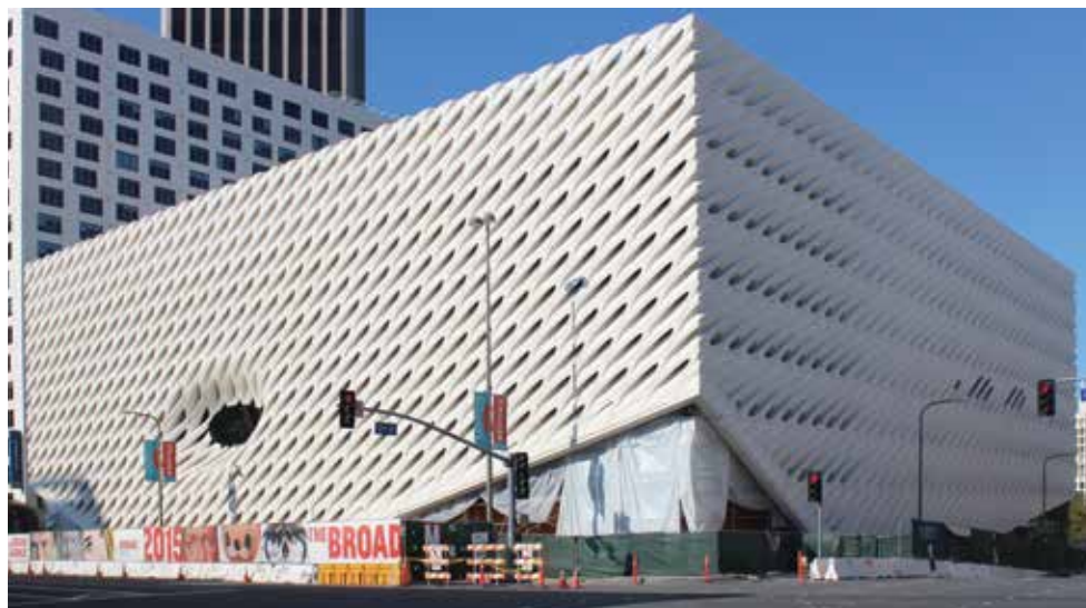
The oculus of the Broad Museum in Los Angeles, Calif., is formed by a depression in the glass-fiber-reinforced concrete panels that penetrates the interior glazing. Courtesy of Willis Construction Inc.
