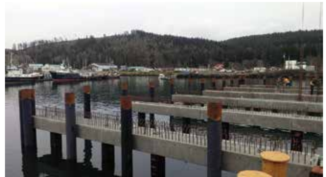
The precast concrete pile caps used in the new Neah Bay fish dock were barged in from Concrete Technology Corp.'s plant in Tacoma, Wash. Courtesy of T. J. Schilling of BergerABAM.
