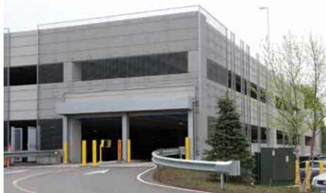
Blakeslee Prestress Inc., the precaster for the new Bridgeport Hospital parking structure in Connecticut, used three-dimensional models to help overcome site challenges. Courtesy of Blakeslee Prestress Inc.
