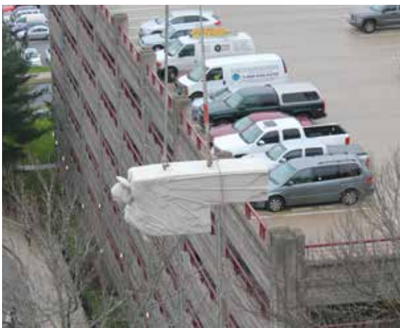
A precast concrete angel flies into place with a little help from a crane. Courtesy of BPDL.
