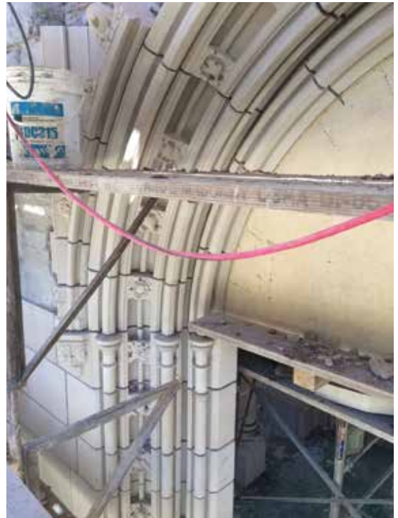
The arch for a window is being assembled. Courtesy of BPDL.
