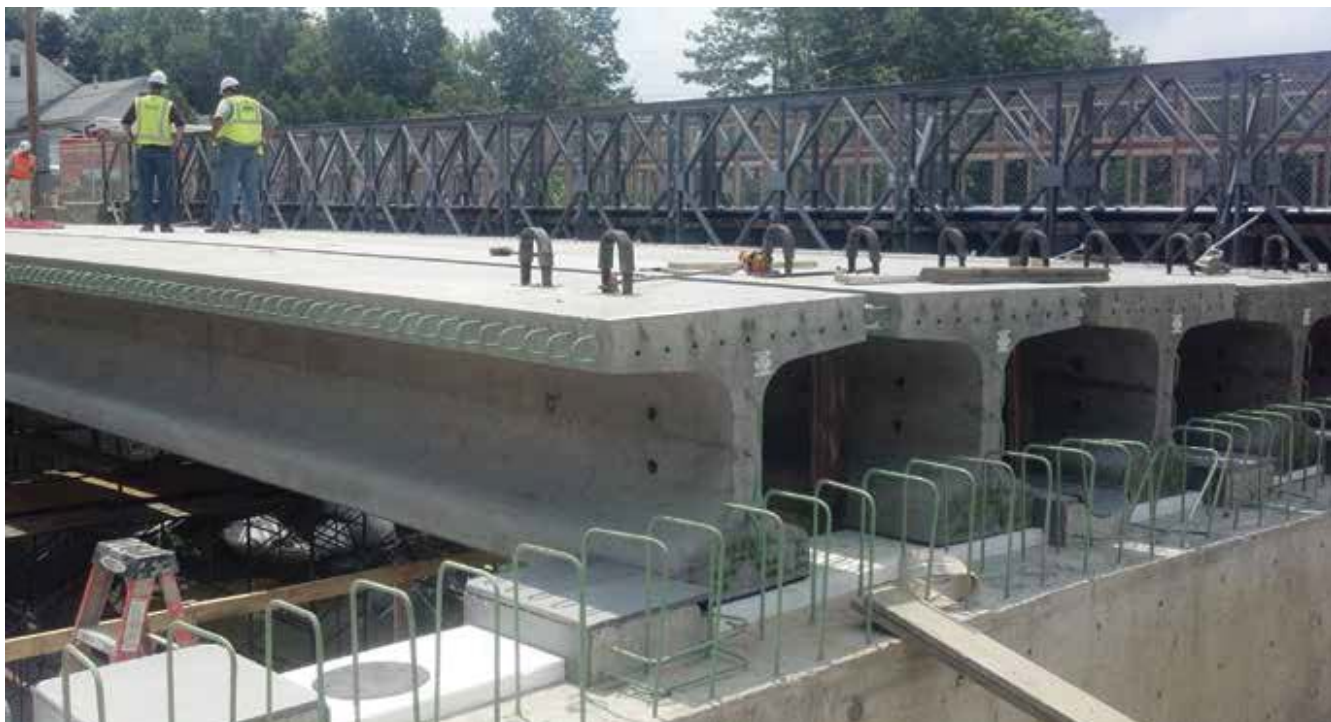
Full deck New England bulb tees are shown on the Manhan River Bridge in Easthampton, Mass. Courtesy of J. P. Carrara & Sons Inc.
