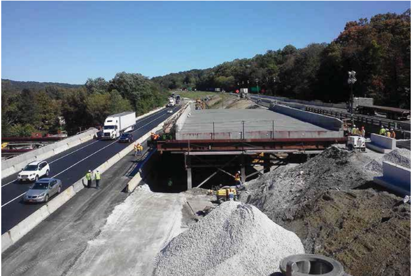
Replacement bridges are resting alongside the existing bridges on Interstate 84 over Dingle Ridge Road in southeastern New York. Courtesy of Dailey Precast.
