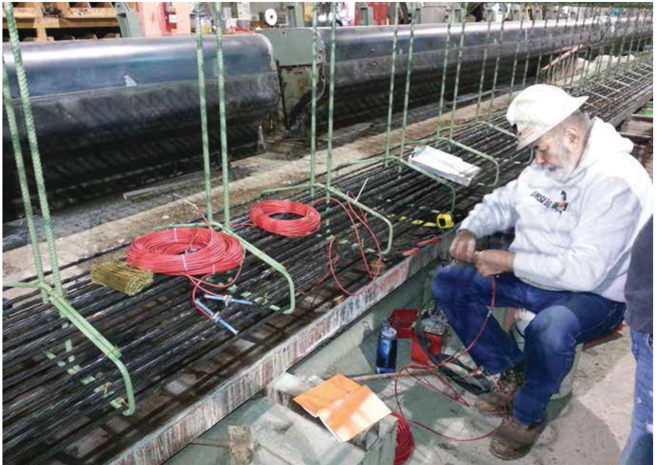
Strain gauges are being installed for long-term health monitoring of the Manhan River Bridge in Easthampton, Mass. Courtesy of J. P. Carrara & Sons Inc.
