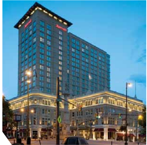
High Concrete Group LLC garnered the grand prize award for architectural concrete/precast concrete cladding from the Eastern Pennsylvania and Delaware chapter of the American Concrete Institute for the Lancaster County Convention Center and Lancaster Marriott at Penn Square in Lancaster, Pa.
