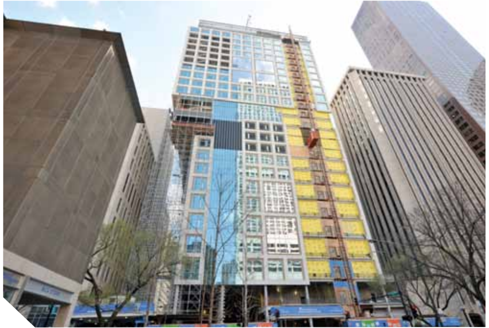
Construction on the Ann and Robert H. Lurie Children's Hospital of Chicago is shown in April 2010. Courtesy of Children's Memorial.
