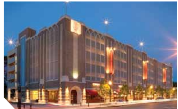
High Concrete Group LLC garnered the grand prize award for precast concrete building systems from the Eastern Pennsylvania and Delaware chapter of the American Concrete Institute for the Saint Joseph's University Hawks Landing Parking Garage in Philadelphia, Pa.
