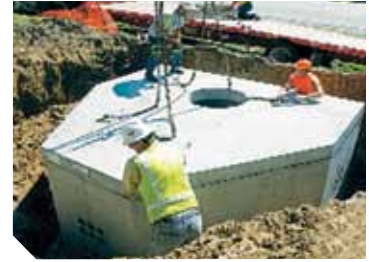
Oldcastle Precast is providing precast concrete manholes, hand holds, and telecommunication shelters to AT&T Government Solutions Inc. at Ft. Leavenworth Army Base in Kansas as part of the Army's $4 billion Infrastructure Modernization Program. Courtesy of Oldcastle Precast Inc.
