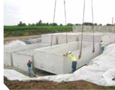
Wastewater holding tanks provided by Oldcastle Precast and part of Oldcastle Inc. are installed in Reynolds, Ind., as part of an algae-based wastewater system that generates power for the wastewater plant. Courtesy of Oldcastle Precast Inc.
