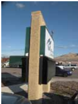
The precast concrete site sign used no portland cement in the mixture.
