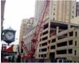
Construction was possible from only one side of the 915 Walnut Street Parking Structure in downtown Kansas City, Mo. Courtesy of Dirk McClure of IPC Inc.
