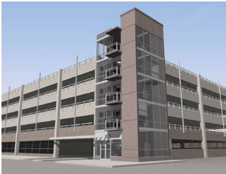
Carl Walker Construction will build a new parking structure for the Pittsburgh Technology Center in Pittsburgh, Pa. Courtesy of Indovina Associates Architects.
