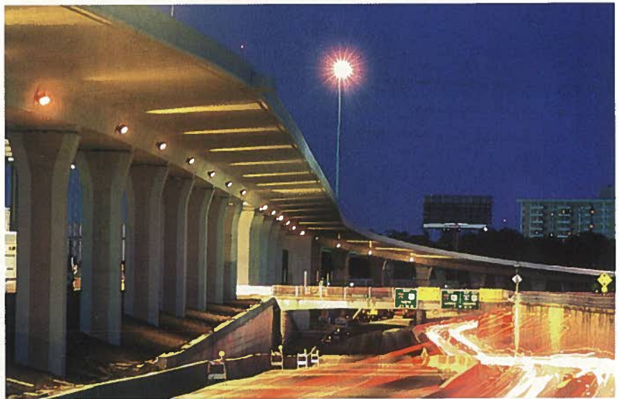
Fig. 12. The San Antonio, Texas, “Y” bridges, built in the existing right-of-way (downtown I-10 and I-35), exemplify the value of precast concrete segmental bridges for construction in extremely restricted urban areas while maintaining traffic flow.
