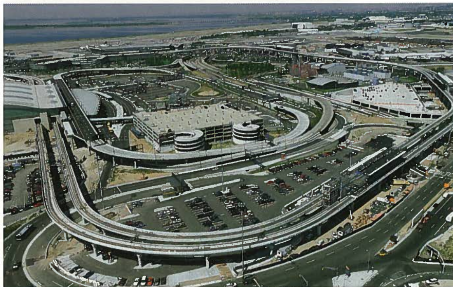
Fig. 17. AirTrain, New York's John F. Kennedy International Airport passenger train, proudly opened 9 miles (14.5 km) of precast concrete segmental bridge transport to the public in 2003. Within the confines of a narrow right-of-way, the AirTrain rises above the six-lane Van Wyck Expressway.
