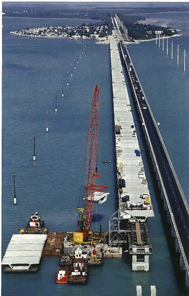
Fig. 2. With the first “as cast” riding surface in the United States, the 2.3 mile (3.7 km) Long Key Bridge in the Florida Keys was completed at a cost of $32.66 per sq ft ($352/m 2 ) in 1980, confirming the economic feasibility of precast concrete segmental technology.
