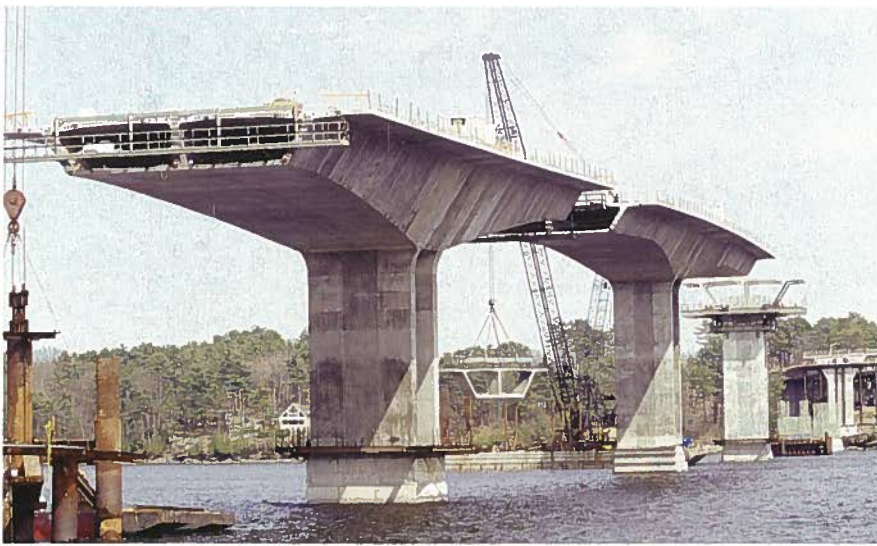
Fig. 9. Sagadahoc Bridge in Maine has a 420 ft (128 m) precast segmental main span and was completed in 2000. Precast concrete segments weighed 100 tons (91 tonnes).
