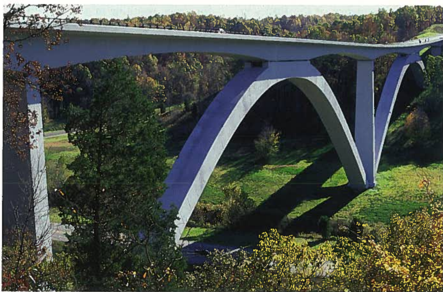
Fig. 6. The impeccably beautiful Natchez Trace Parkway Arches is America’s first use of precast concrete segmental technology for an arched structure. It was completed for $11.3 million in 1994.
