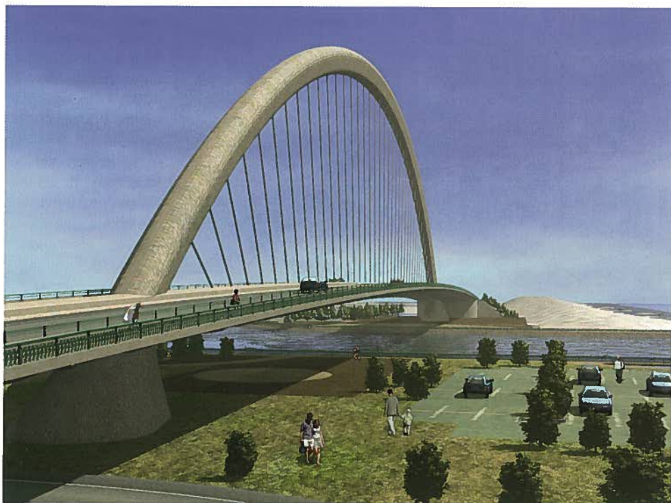
Fig. 22. An artist's rendering of the proposed Indian River Inlet Bridge, in Delaware's Seashore State Park, captures the intrinsic beauty of a 1000 ft (305 m) precast concrete arch cable-stayed span.
