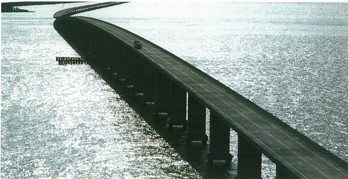
Fig. 3. The longest continuous precast segmental bridge in the world in 1982, the Seven Mile Bridge in the Florida Keys was the first use in North America of precast, match-cast box piers, assembled with vertical post-tensioning.
