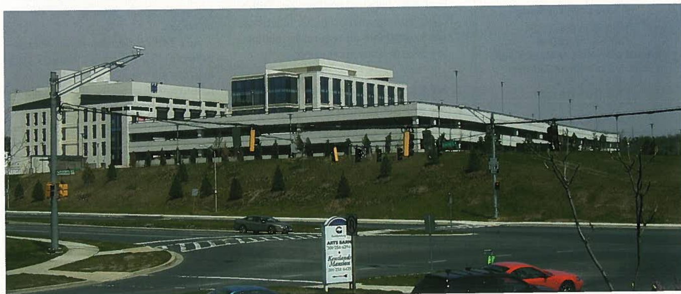
Overview of new parking structure in front and the medical facility in back.
