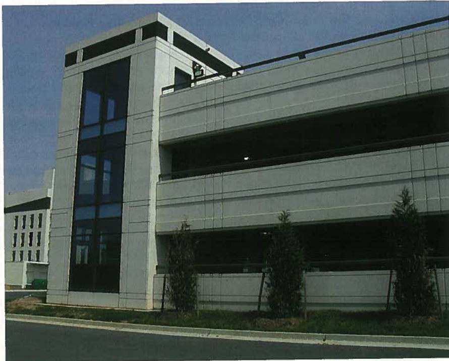
Closeup of parking structure showing the architectural precast, spandrel panels with a light sand-blast finish. Recessed areas and reveals provide relief and interest to the panels that wrap the massive structure.
