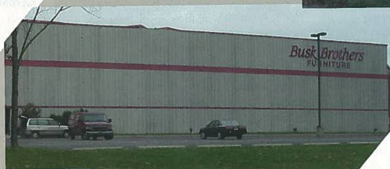
Fig. 3. Busk Brothers Building (Building B).
