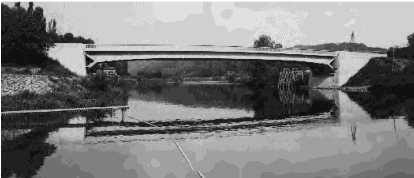
Fig. 4. Luzancy Bridge across the Marne River, France (1946). This elegant bridge (designed and built by Freyssinet) was the first major bridge in the world built of precast, prestressed segmental construction.
