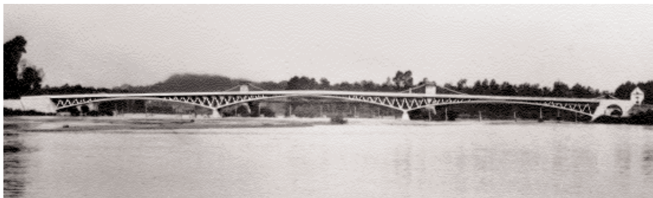
Fig. 1. Le Veudre Bridge across the Allier River, France (1910-1911). Spans were 222 – 238 – 223 ft (67.5 – 72 – 67.5 m). This bridge incorporated the first use of thrust by jacks at midspan for decentering and also compensating for concrete creep and shrinkage. (Designed and built by Eugene Freyssinet.)
